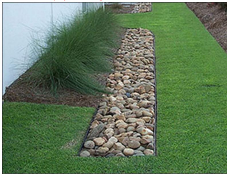
Image 7: Typical Infiltration Trench similar to that proposed for the housing units within the Barnhill SHD
