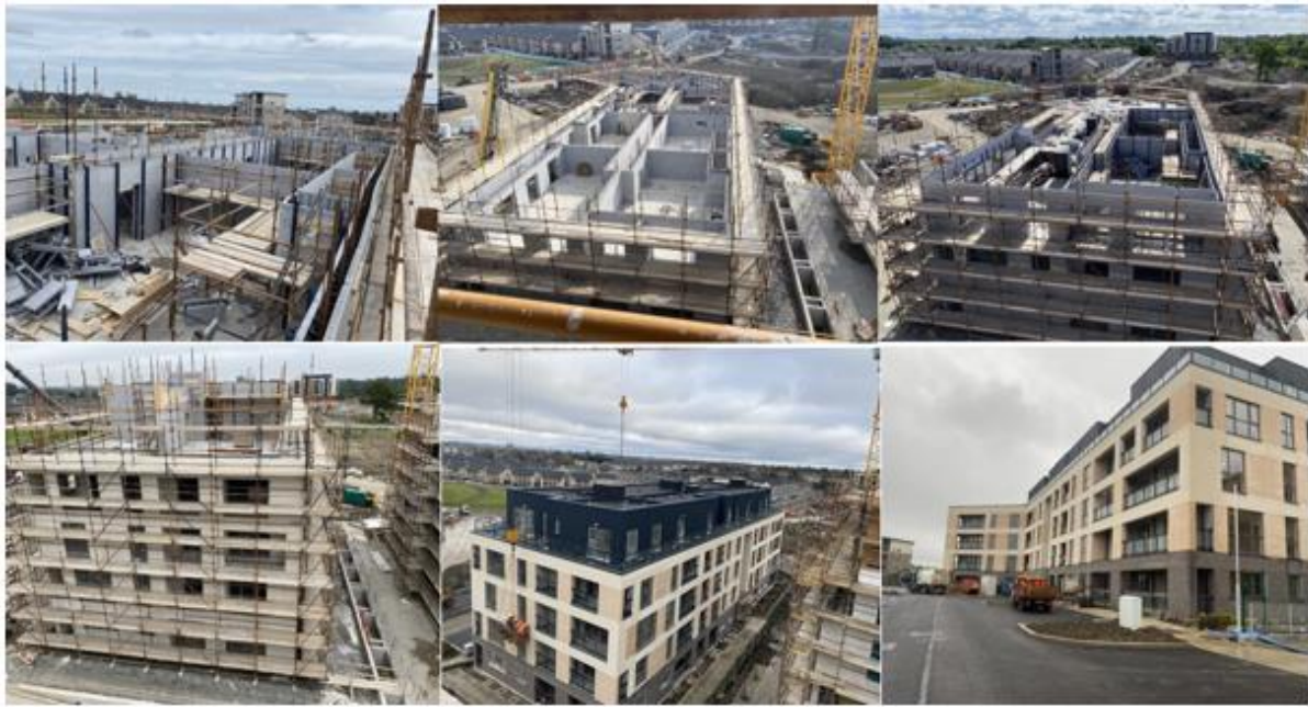
Figure 6: Apartment Block Construction in ICF
