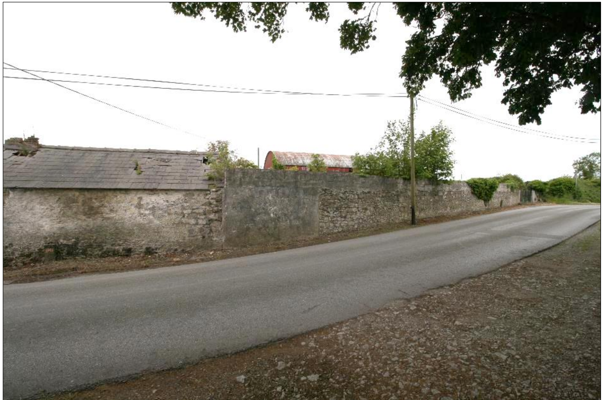
Plate 13.2.3: Random rubble masonry boundary wall (raised with concrete blocks) which formed rear wall of now-demolished building attached to west gable of ruined, but upstanding former dwelling (slate roof to left side of photograph).
