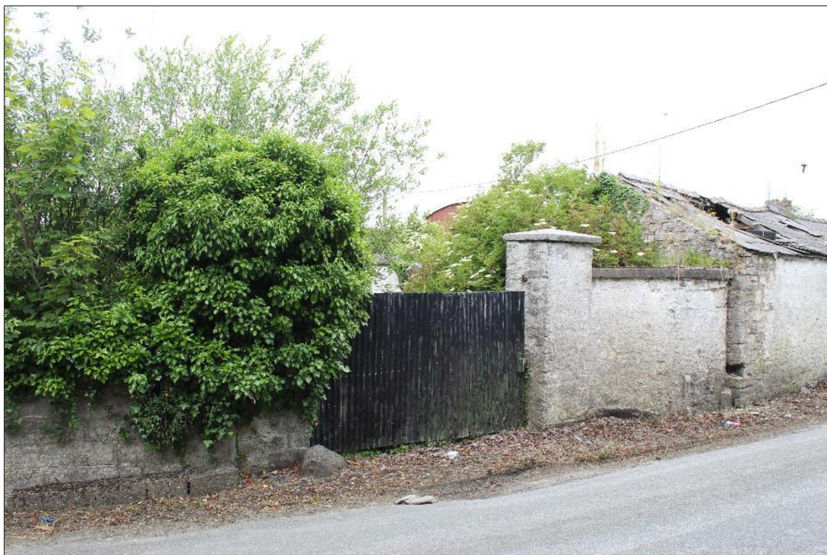
Plate 13.2.2: Square masonry gate piers with pyramidal granite caps, replacement wrought-iron gate and curved masonry wing wall on west (right) side (; concrete blocks abut east (right) pier). Gateway leads to vernacular, formerly residential farmyard which predates mid-later nineteenth-century Barnhill House
