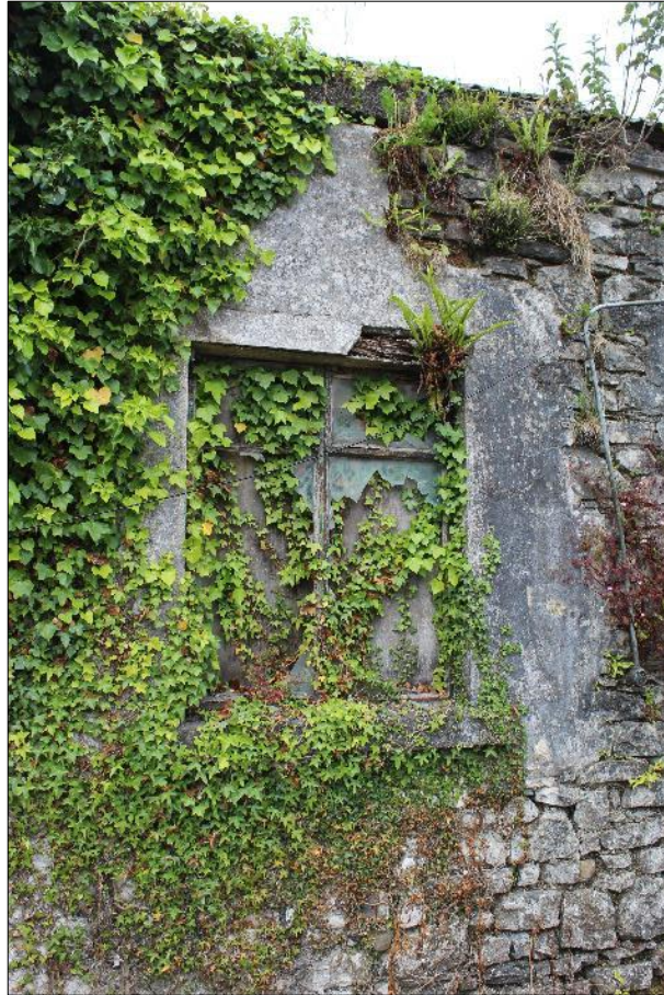
Plate 13.2.13: Inserted steel-framed window and concrete surrounding infill in rubble masonry wall of taller farm building opposite former dwelling
