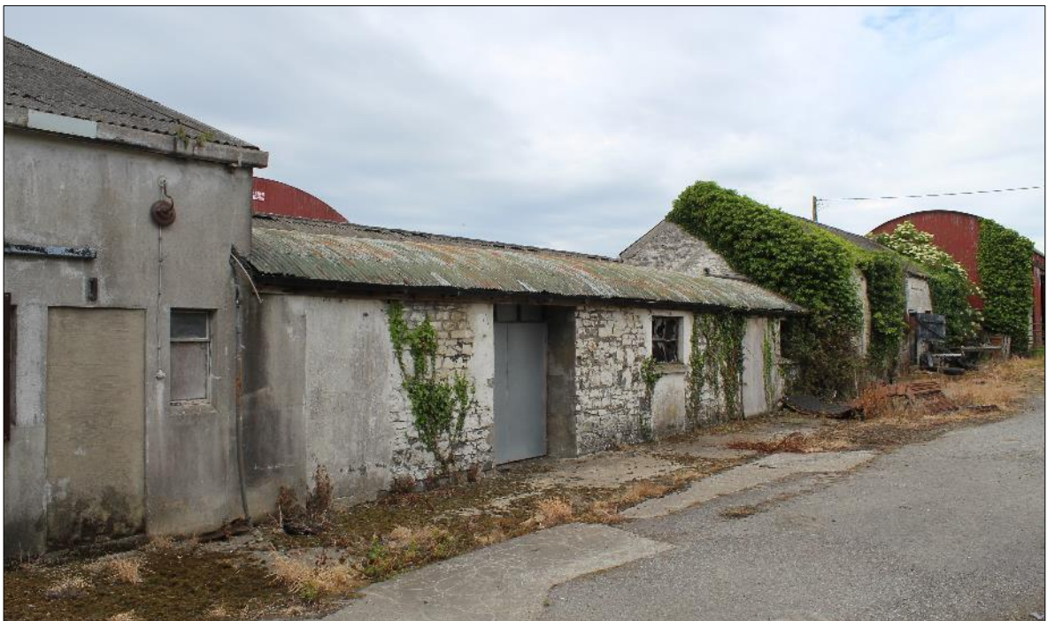
Plate 13.2.10: Altered north-east elevation of historic farm building. Profile of former pitched roof of this building visible on south-east gable of adjoining taller building which is directly opposite façade of former dwelling.
